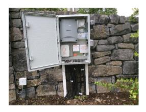
Our complete enclosure to house all electronic control units including main power isolator, mains circuit breakers, gate/barrier/bollard control panel, loop detector, GSM control unit, app control unit and override switch for safety photo sensors.
